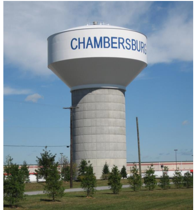
Figure 4: Nitterhouse Drive Elevated Composite Tank
