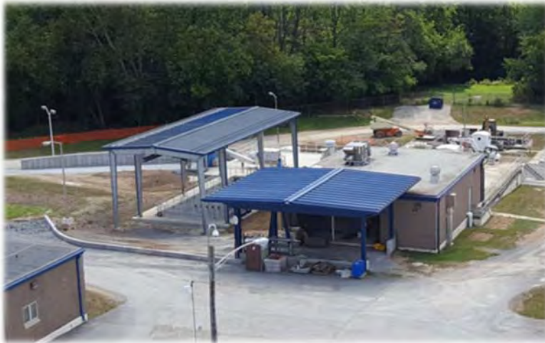
New Influent Pump Station (Headworks)
