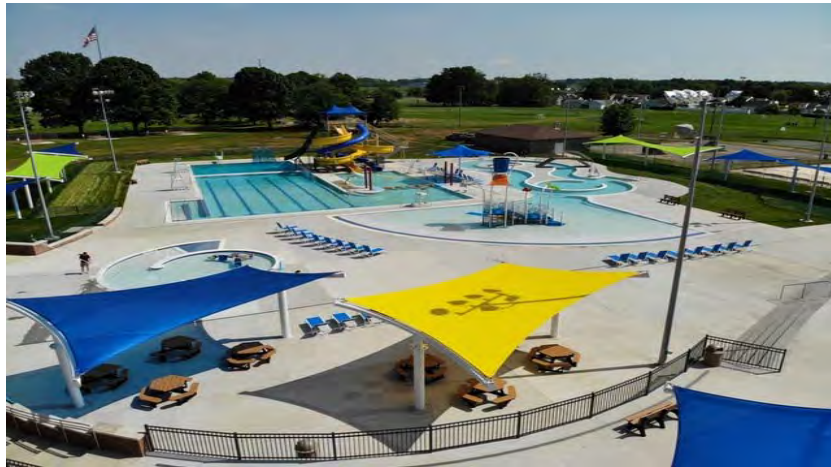
The Finished Facility 2018
