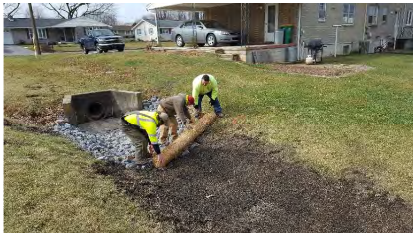
Highway Personnel Help with a Storm Water Project
