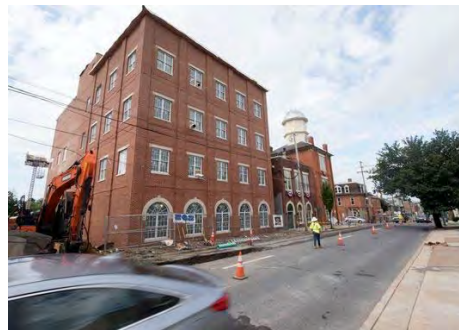
The Utility Departments' Addition for City Hall under construction in 2018
