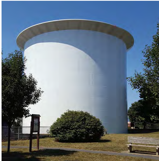
Birkinbine Tank was Re-Painted in October 2015
