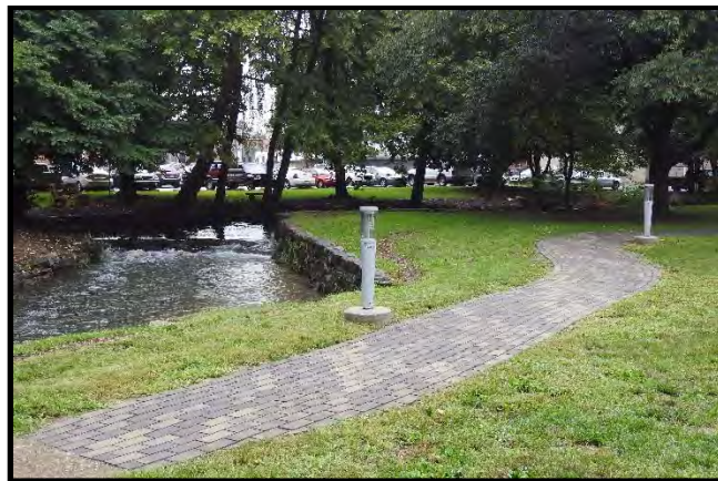
New Pedestrian Walkway as a Part of Rhodes Drive BMP Project
