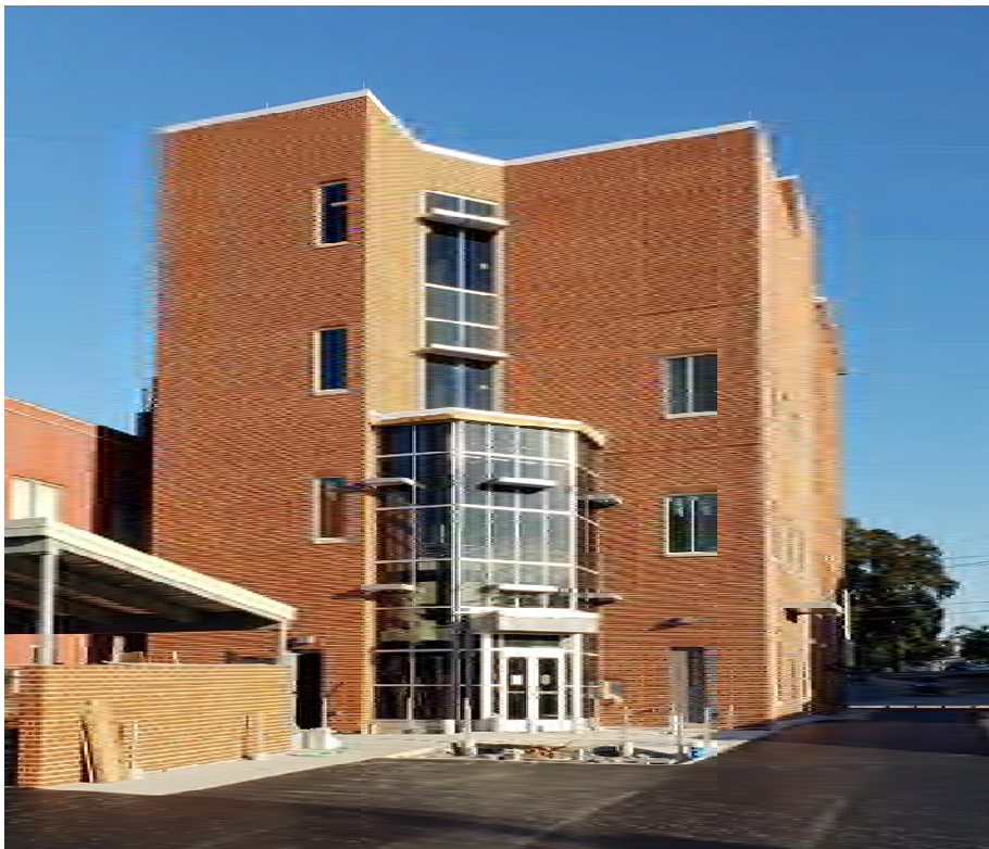
Building Exterior Nearing Completion
