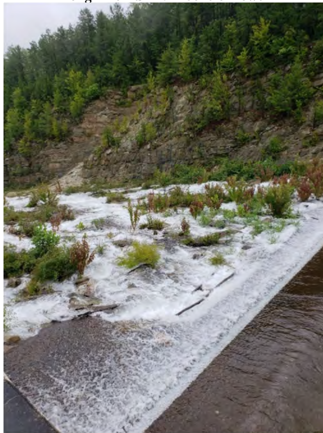
Long Pine Spillway – July 2018
