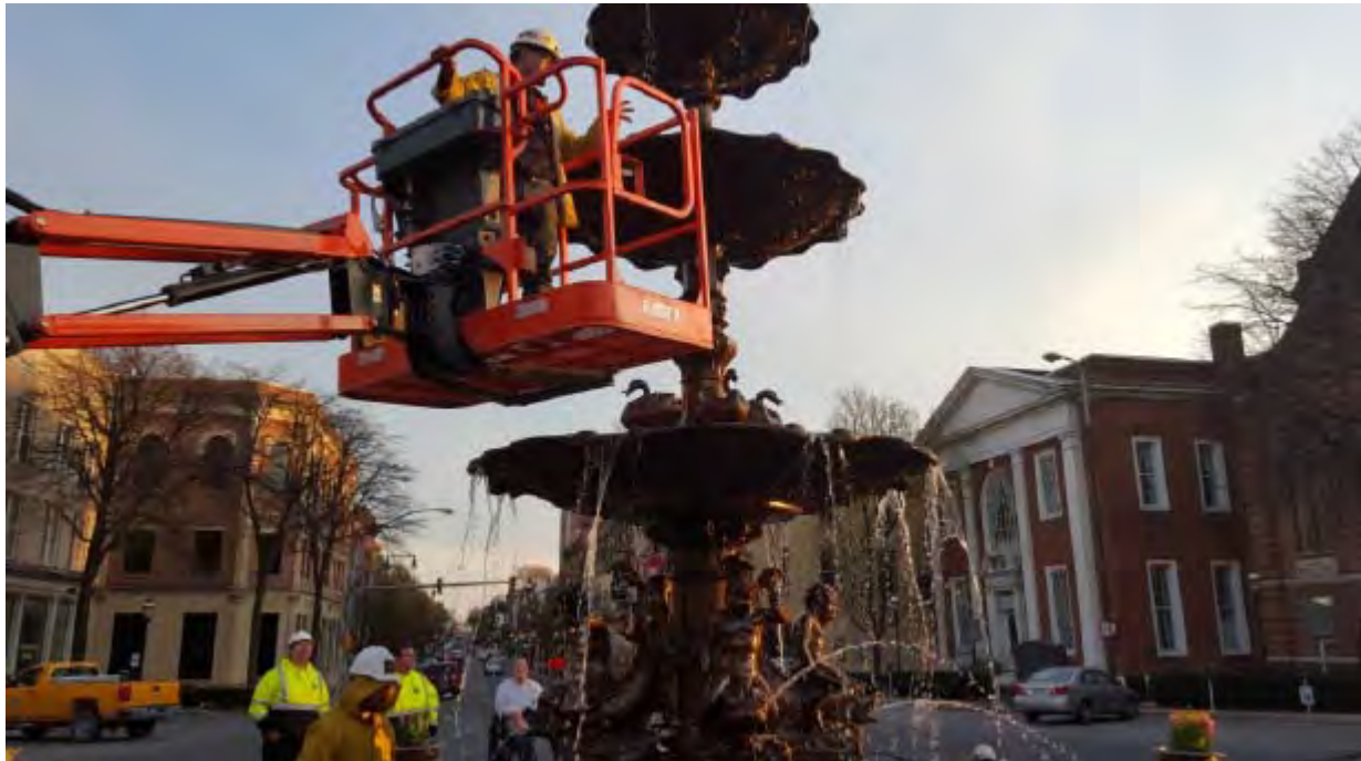
Maintenance of the Memorial Square Fountain
