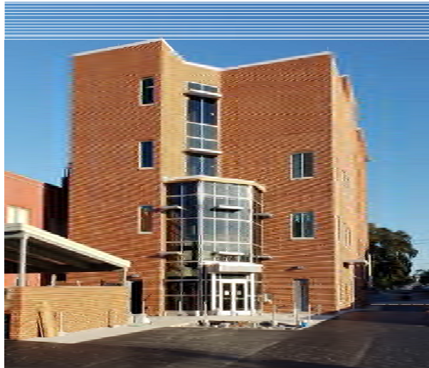
Building Exterior Nearing Completion
