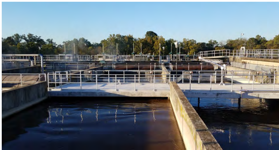
Modified VLR Tanks in Operation in 2017
