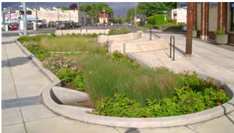
Example of Stormwater Best Management Practice (BMP) on Private Property
