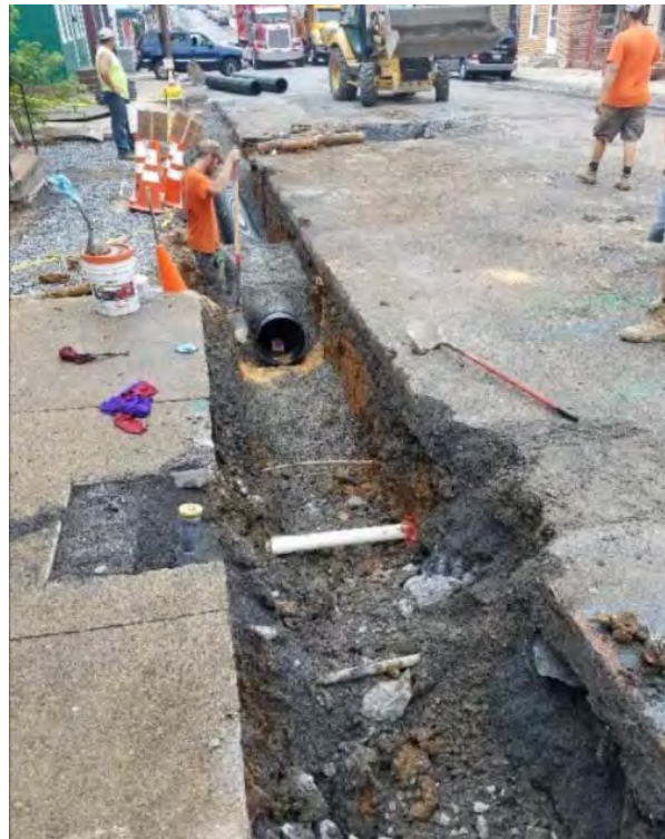
In 2017, storm sewer pipe was replaced on Catherine Street
