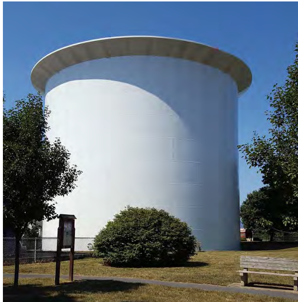
Birkinbine Tank was Re-Painted in October 2015
