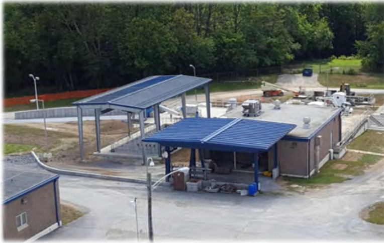
New Influent Pump Station (Headworks)
