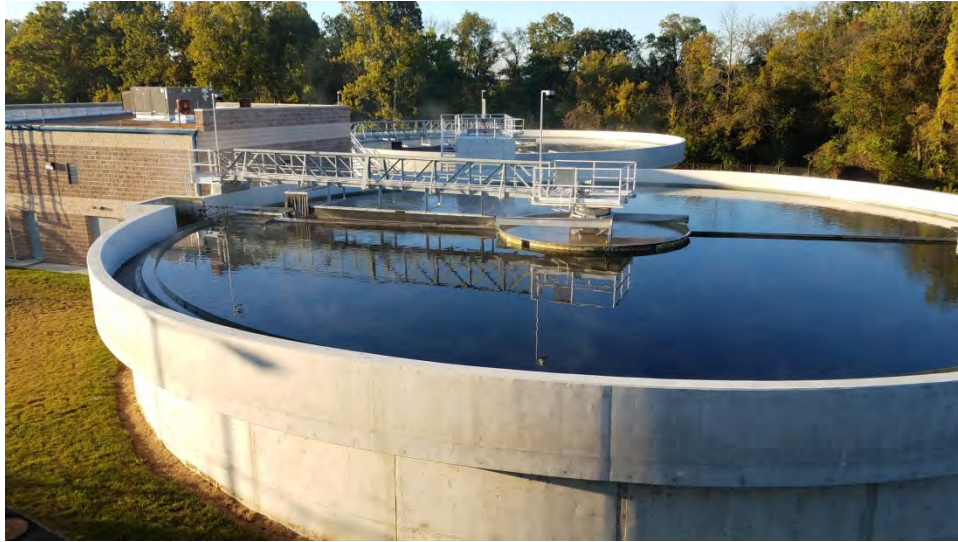
New Clarifies in Operation in 2017
