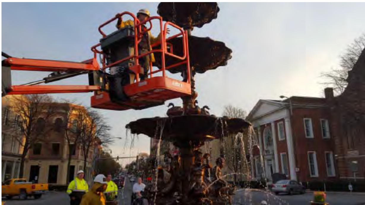
Maintenance of the Memorial Square Fountain
