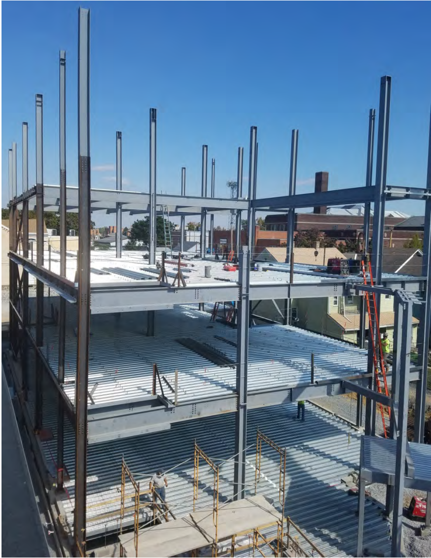
Steel Erection Taking Place for City Hall Addition
