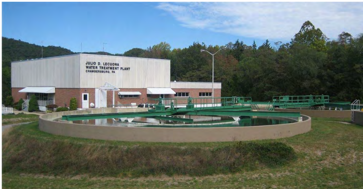
Julio D. Lecuona Water Treatment Plant Greene Township 6.0 Million Gallons Per Day Capacity
