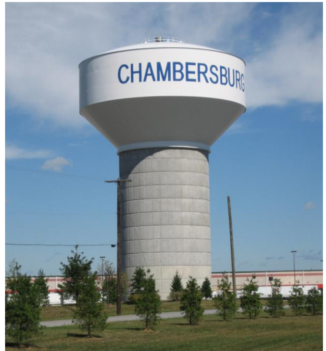
Figure 4: Nitterhouse Drive Elevated Tank
