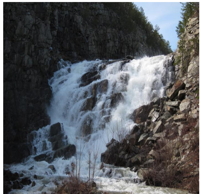
Figure 1: Long Pine Run Reservoir Spillway
