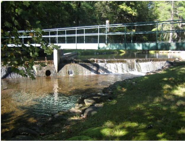
Figure 3: Conococheague Creek Intake Facility
