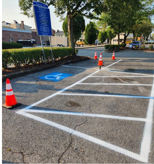
Installing Handicap Parking Stall
