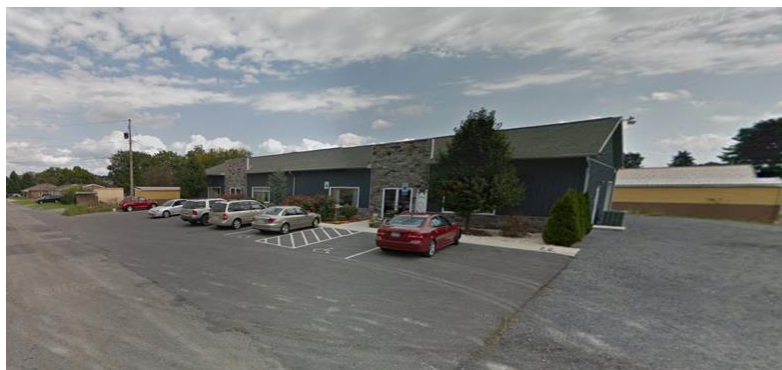
Water/Wastewater Utility Office Building Occupied at 1332 S. Fourth Street
