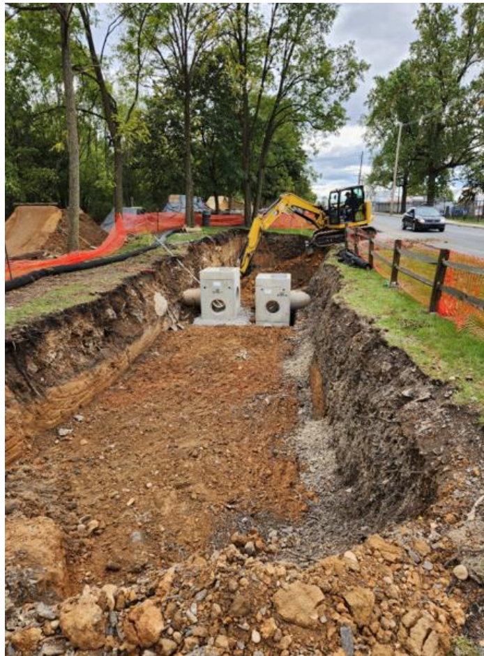
Chambersburg Rail Trail Stormwater Improvement
