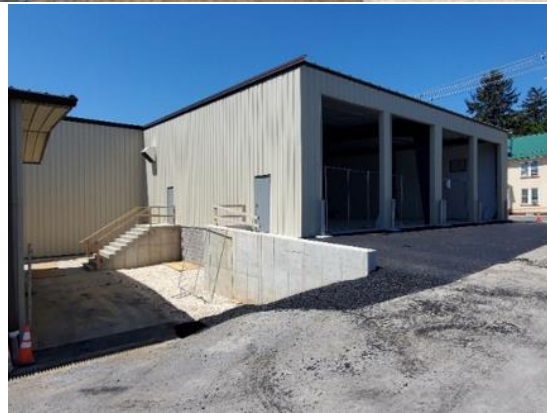
Rear Line Truck Bays – New Electric Distribution Operations Center
