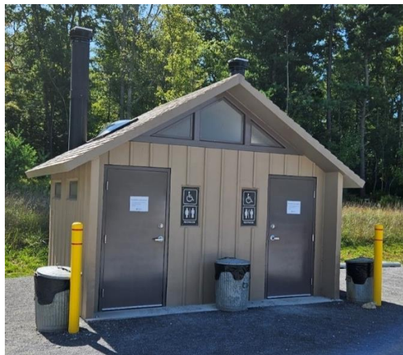
Long Pine CXT Restroom – Summer 2024
