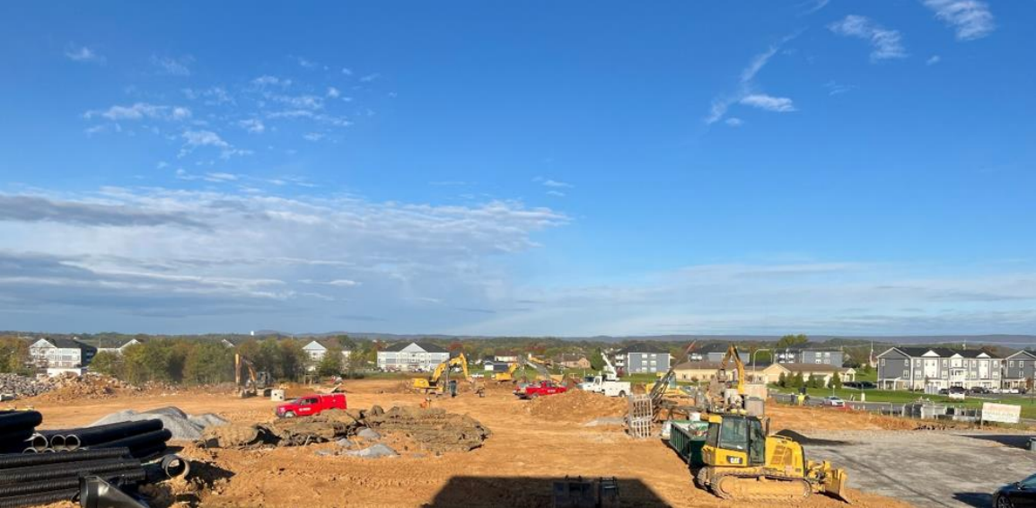
Orchard Drive Apartment Complex Under Construction
