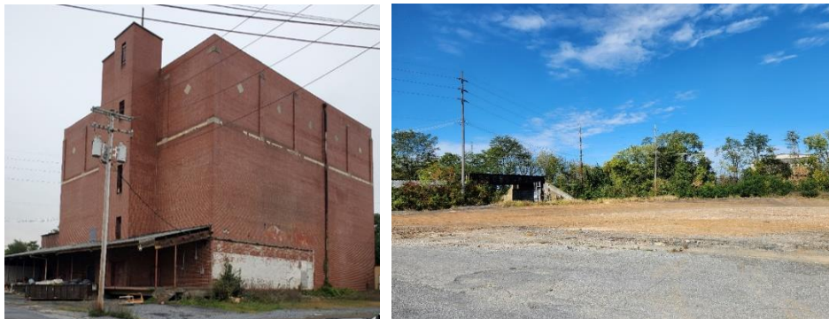
Old Cold Storage Building on S. Fourth Street – Before and after demolition
