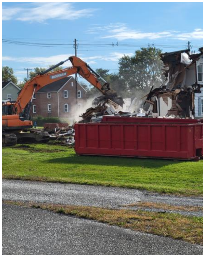
Demolition of Previous Properties Underway in 2024
