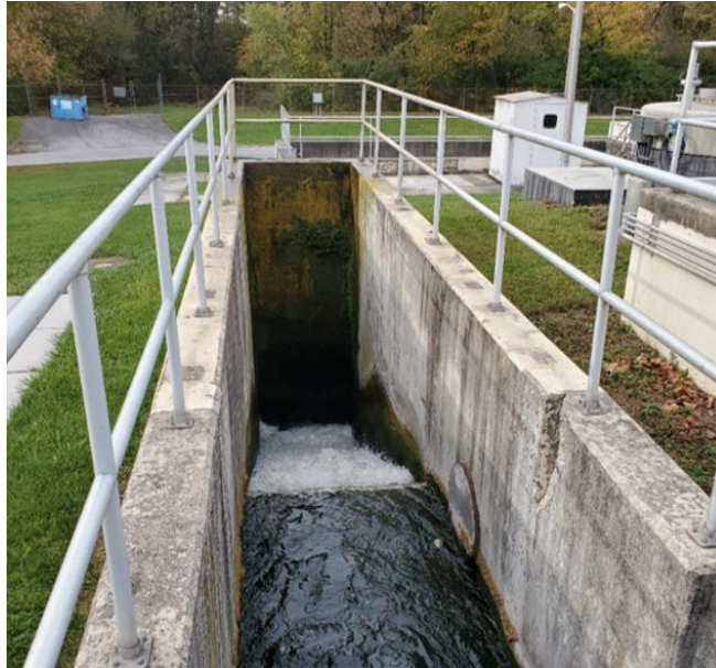
Final Outfall to Conococheague Creek
