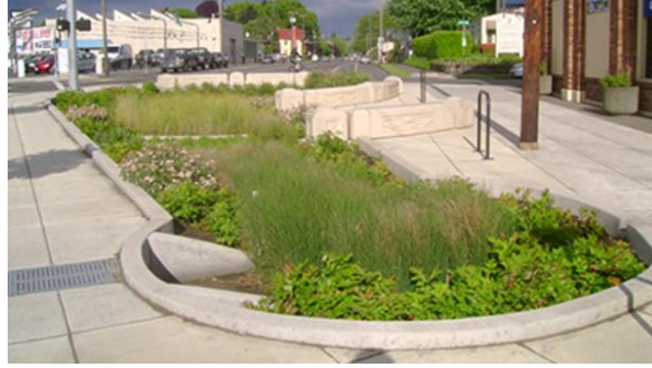
Out-of-Town Example of Stormwater Best Management Practice (BMP) on Private Property
