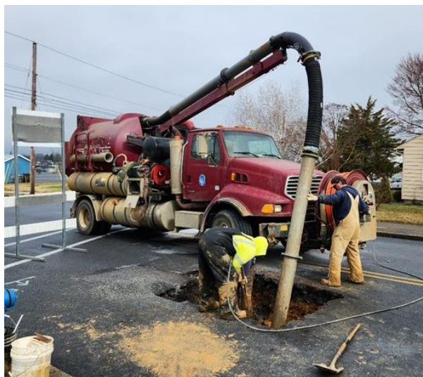
Water Service Excavation with Vac Truck
