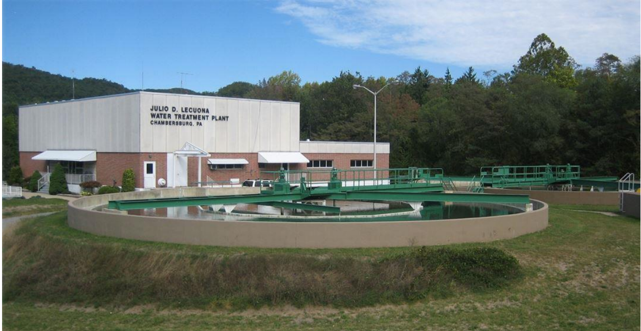
Julio D. Lecuona Water Treatment Plant Greene Township 6.0 Million Gallons per Day Capacity
