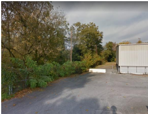
Pump Station Location - Chambers Street
