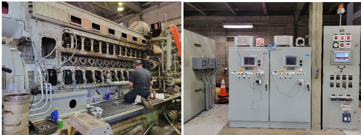
Falling Spring Generation Station – Engines, Controls, and Renovations 2021-2022
