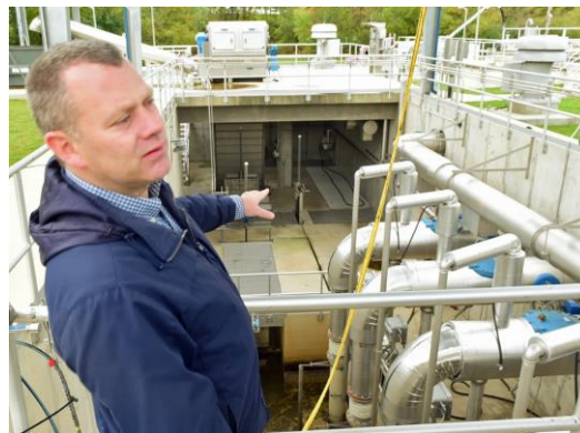
Lance Anderson at the Headworks
