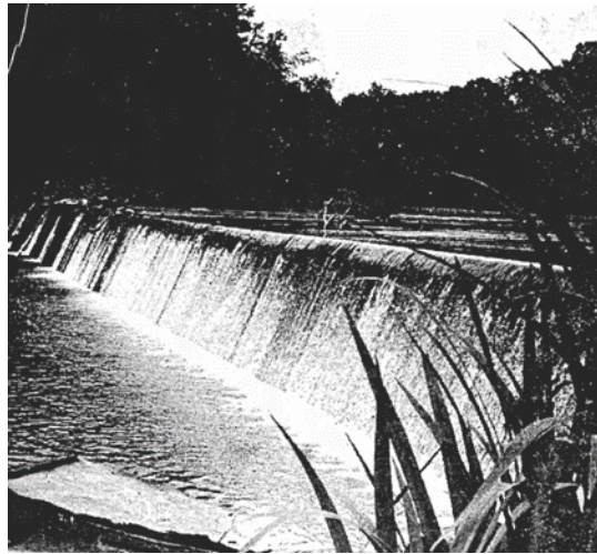
The Second Siloam Dam
