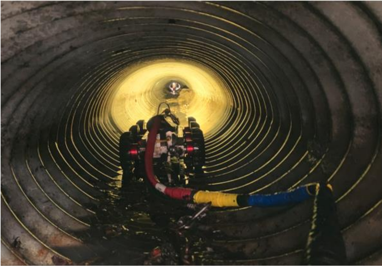
Storm Sewer Pipe Cleaning and CCTV Recording Project
