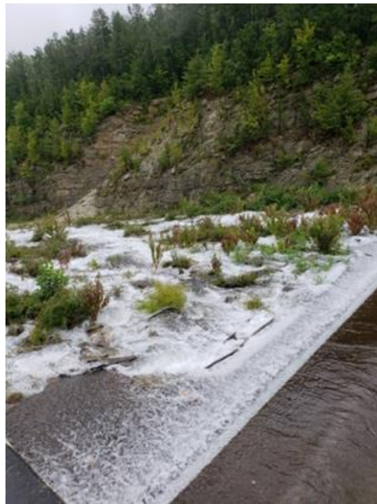
Long Pine Spillway – July 2018
