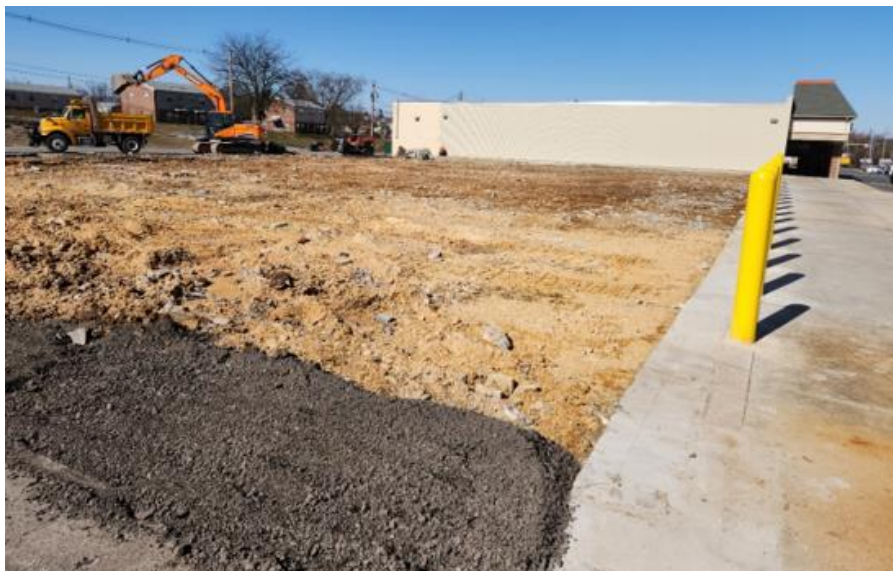
Building a Temporary Parking Lot at the Southgate Shopping Center
