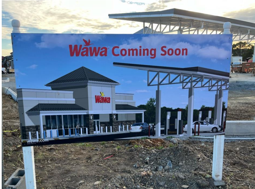
Wawa Convenience Store Under Construction on Wayne Avenue
