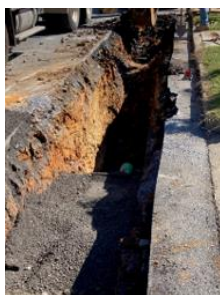
Sewer Main Installation
