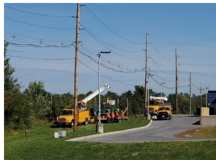
Line Crews Installing Underground Cable & Overhead Messenger for Fiber Network
