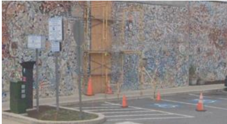
One of two existing parking kiosks in the Rosedale Parking Lot
