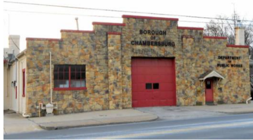
Existing public works facility on Loudon Street dates from the beginning of the last century
