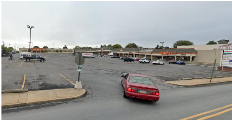
The dilapidated half-empty Shopping Center as it appeared in 2022
