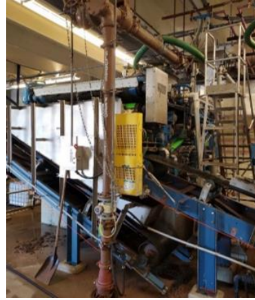
Aging Equipment – Belt Press
