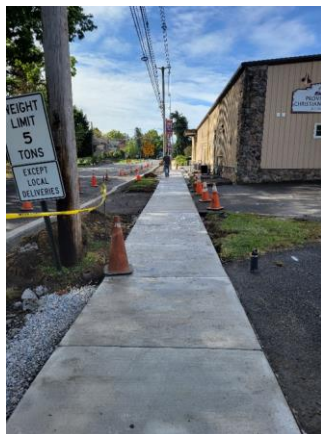
5th Avenue & Grant Street – Curb and Sidewalk Installation
