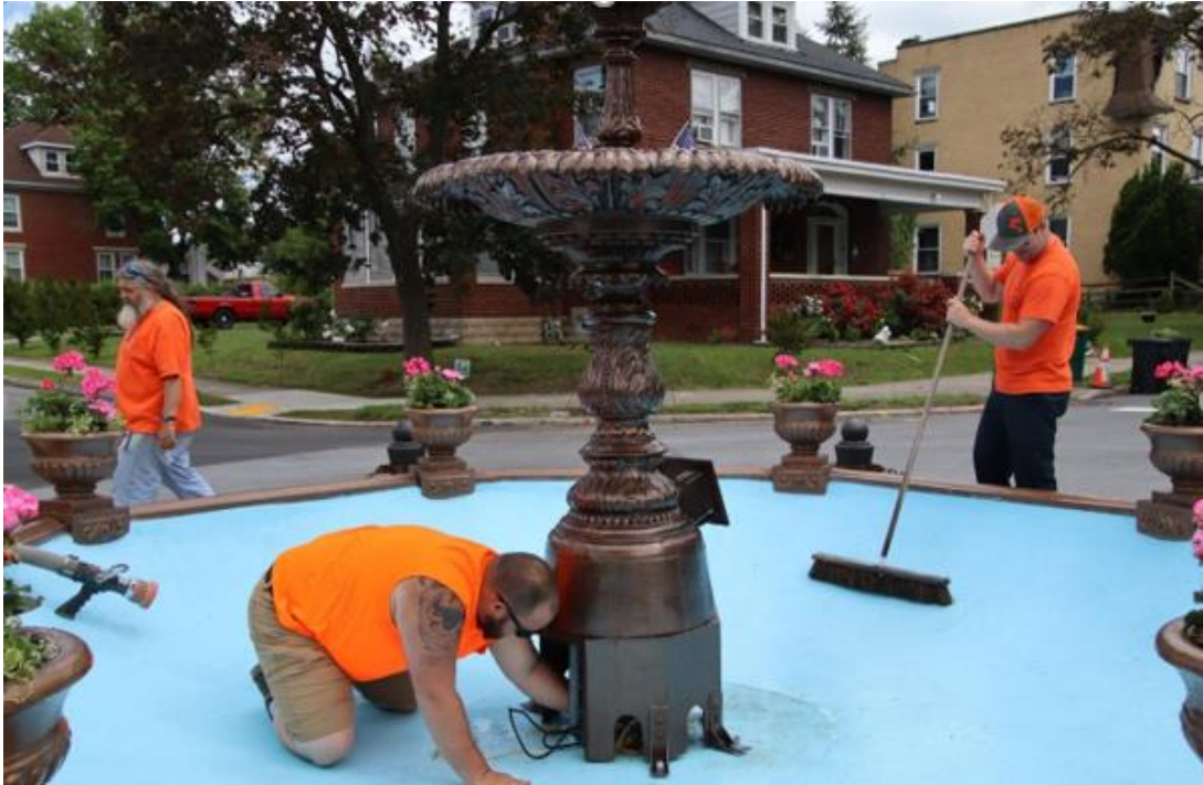
Reinstallation of the Refurbished Glenn Street Fountain
