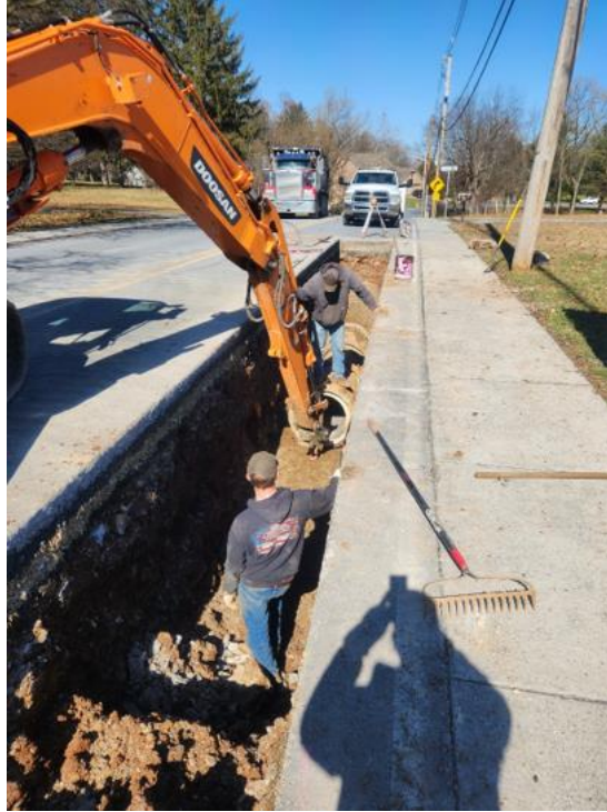
Limekiln Drive Pipe Replacement
