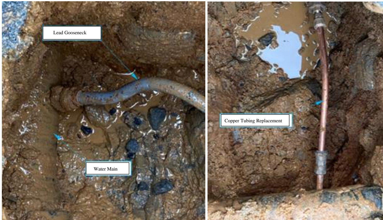
Water Service Before Gooseneck Removal - Water Service After Gooseneck Removal
