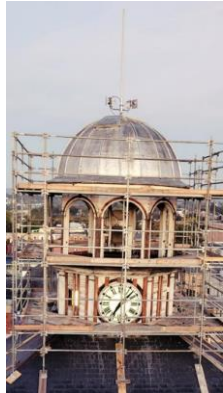
Clock Tower being restored in 2022
