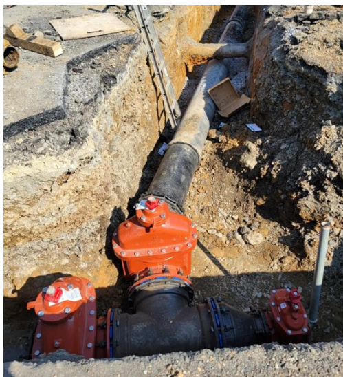
Chambers Street/Reservoir Hill Water Main Extension
