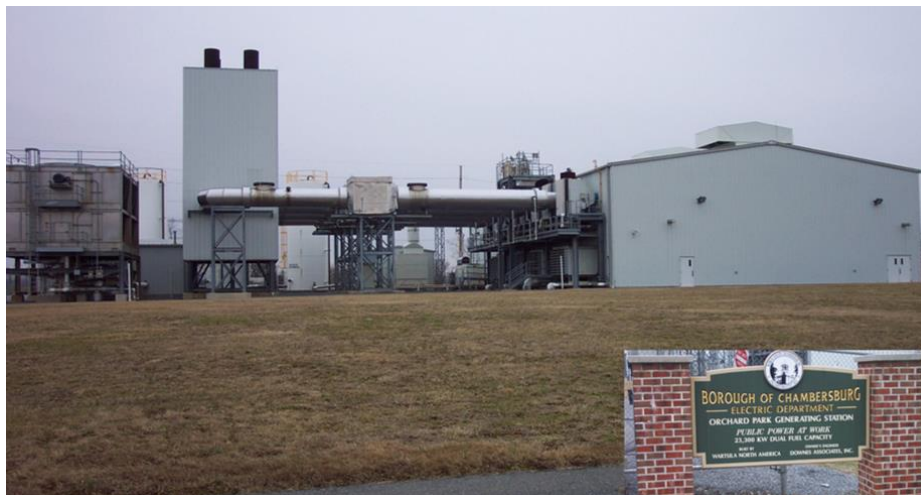
Orchard Park Generating Station
