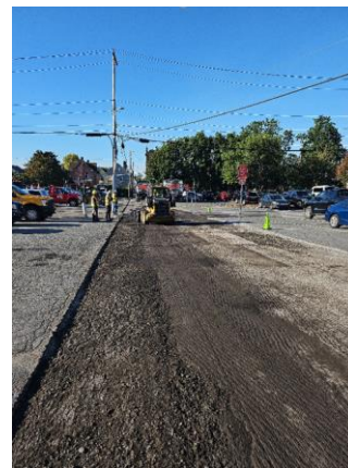
Paving Operation – S. Harrison Avenue & E. Ludwig Avenue
