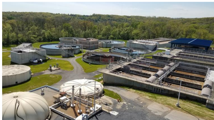
J. Hase Mowrey Regional Wastewater Treatment Facility
