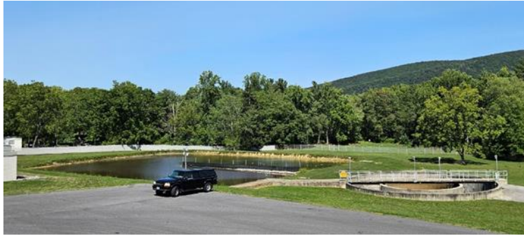
Water Treatment Plant Waste Processing Facilities
